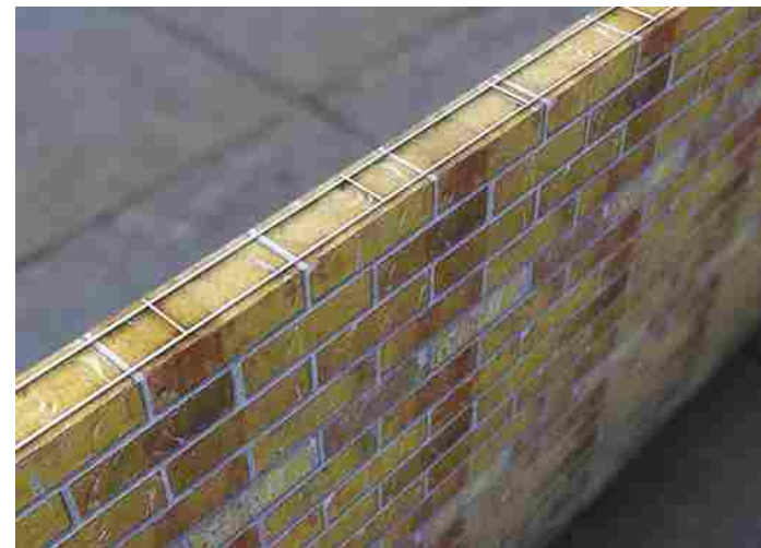
Welded ladder type Bed Joint
